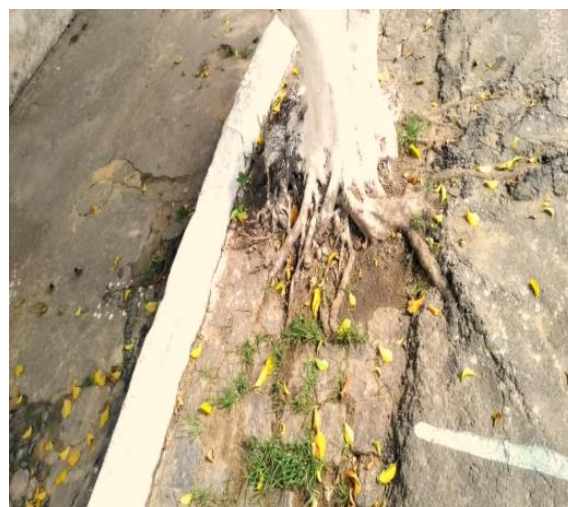
Photo 3. Cracks in the sidewalks and asphalt, caused by the roots of the trees. Photo 4. Cracks in the sidewalks and asphalt, caused by the roots of the trees.
